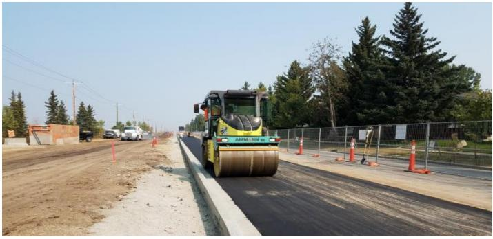
Following the completion of splice vault and duct bank installation, excavated areas will be restored.
