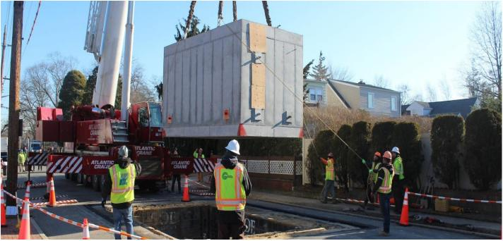
Underground vaults will be installed at intervals along the route to splice, or tie together underground cables.
