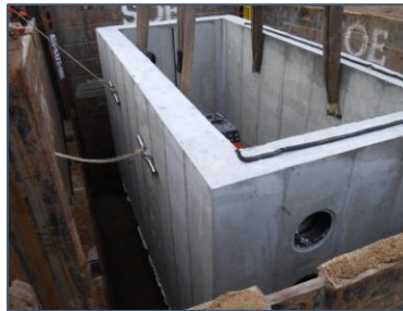
Vault Installation
